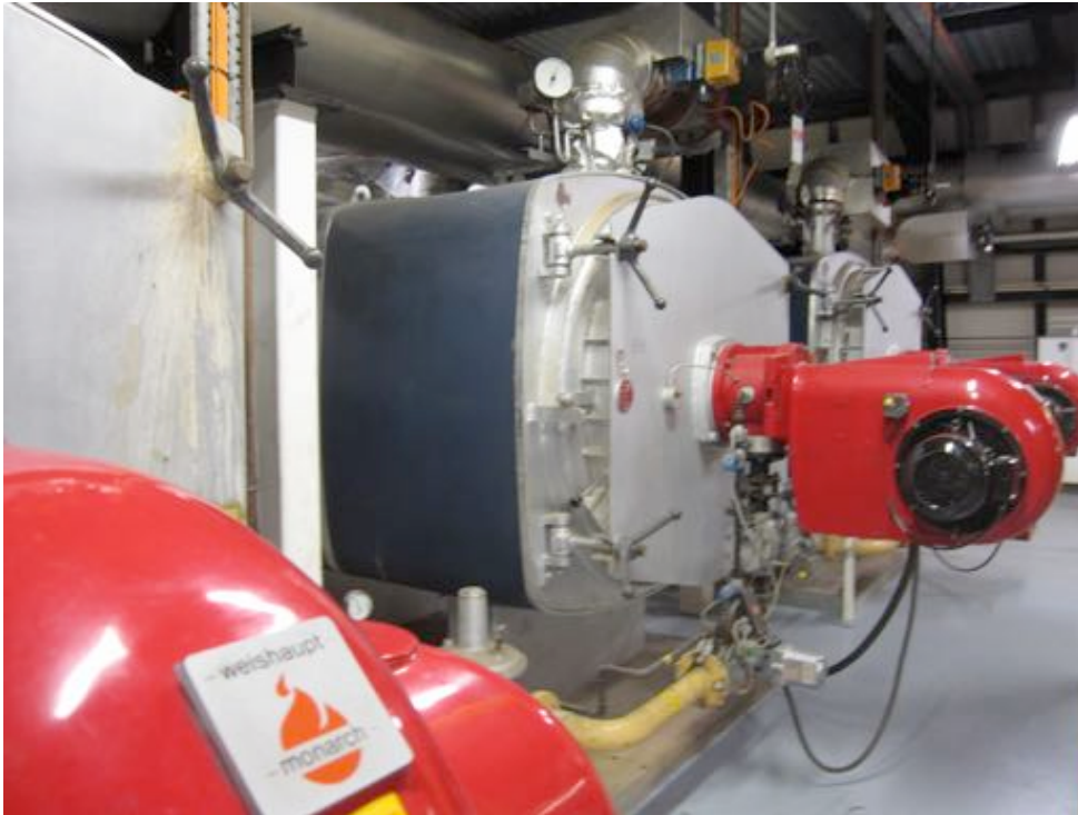
Figure 8.2, Centralised Packaged Boilerroom
