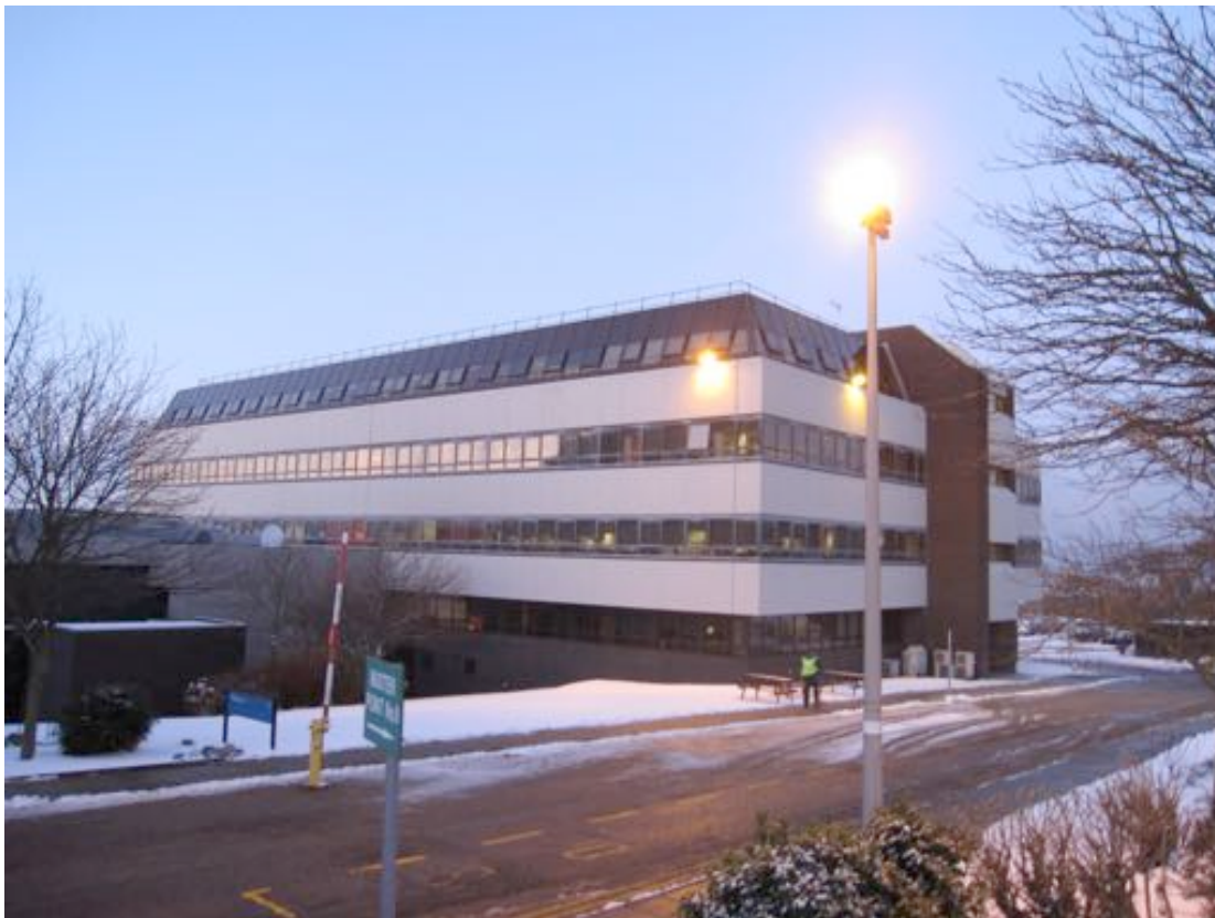
Figure 8.1 – Phase Four, but a similar style to other office accommodation at the site
